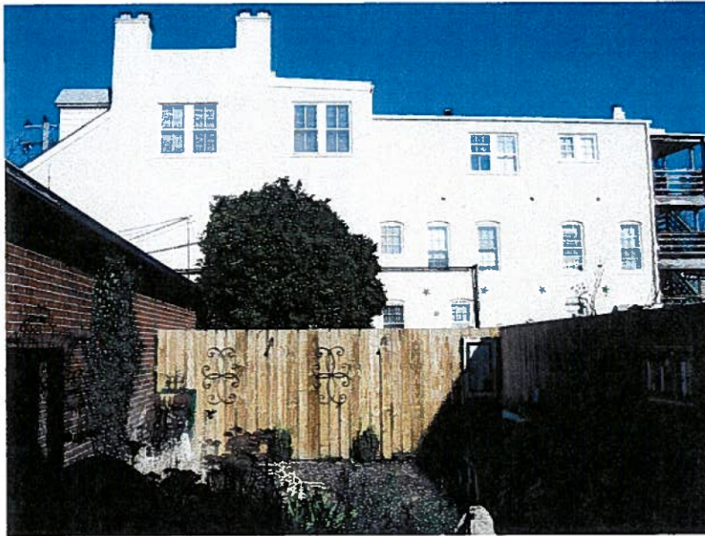
View of rear yard taken from rear of house (facing North)
