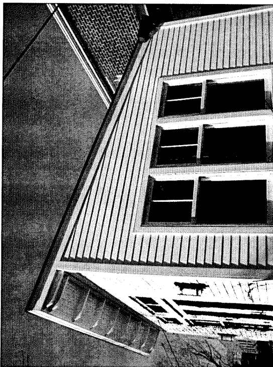
EXISTING ONE-STORY ADDITION
