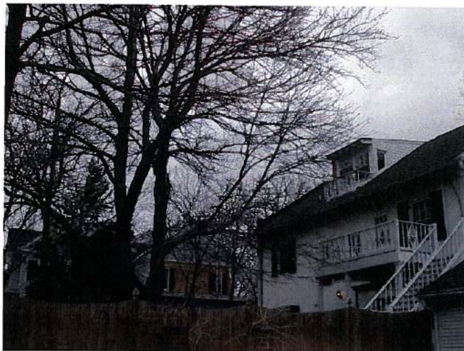
Rear View & Yard
