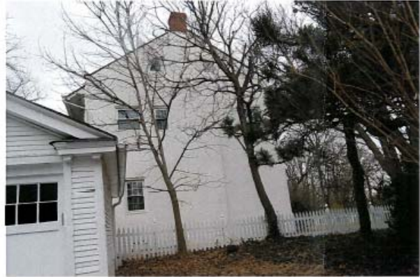
View 4 Side of House, South *Area of special exception
