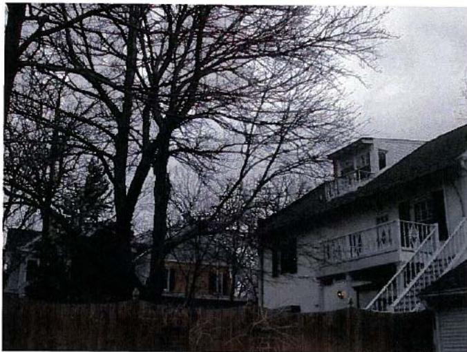
Rear View & Yard
