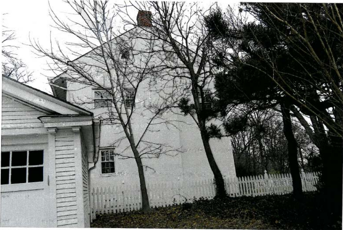
SOUTH ELEVATION OF SUBJECT PROPERTY FROM ADJACENT PROPERTY; NEIGHBOR'S NON-COMPLYING GARAGE SHOWN IN FOREGROUND
