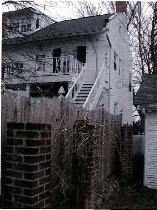
Side & Rear View Of House next to Fence (Property Line)
