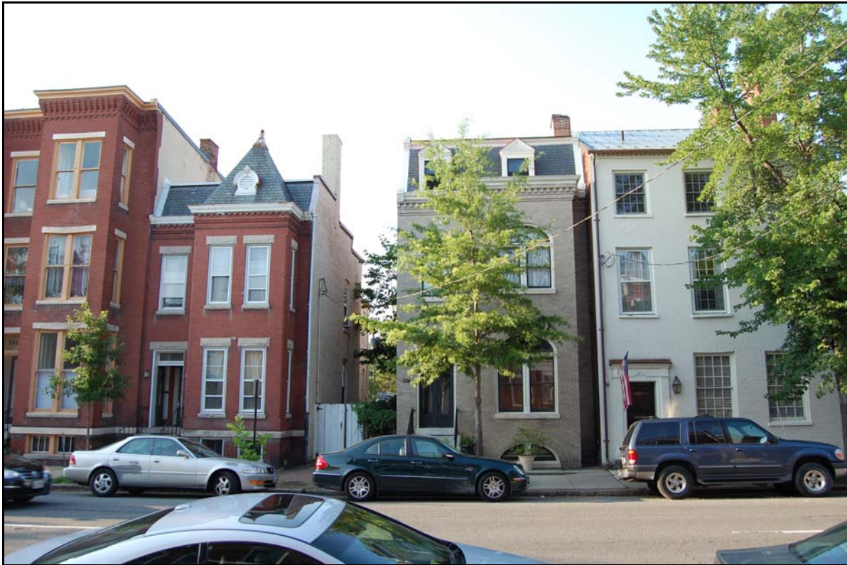
Figure 1 - 911, 909, 907 and 905 Prince Street
