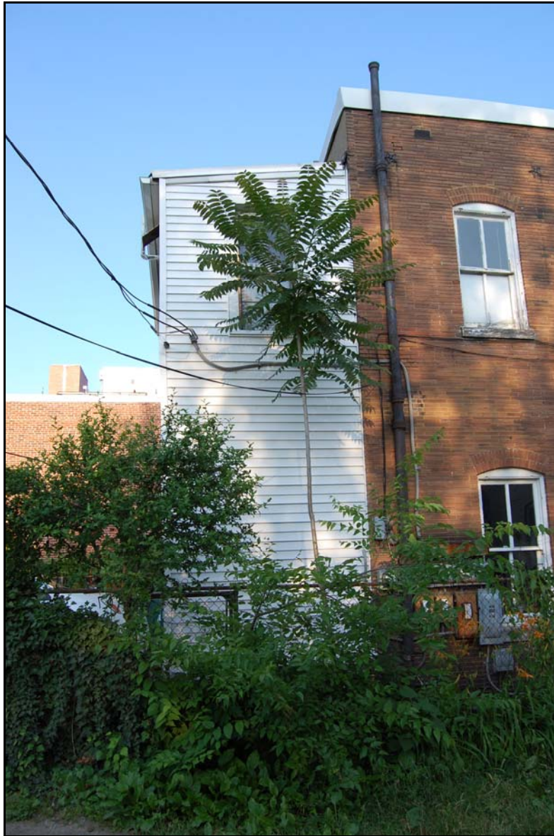
Figure 6 - 907 Prince St rear addition west elevation
