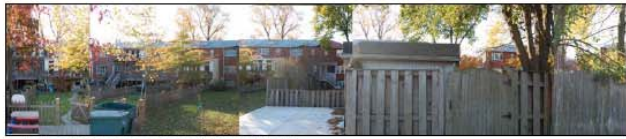
REAR OF 300 BLOCK OF EAST MASON AVENUE VIEW LOOKING SOUTH ALONG ALLEY
