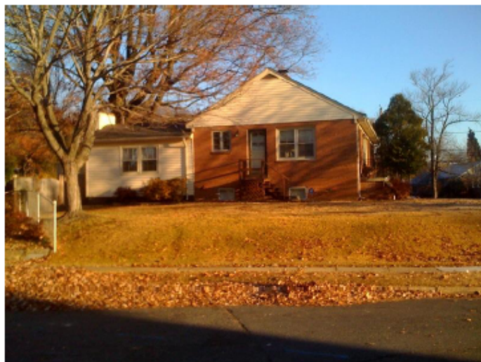
SIDE facing Torrey Place
