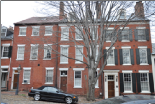
View 6: View across Prince Street facing North
