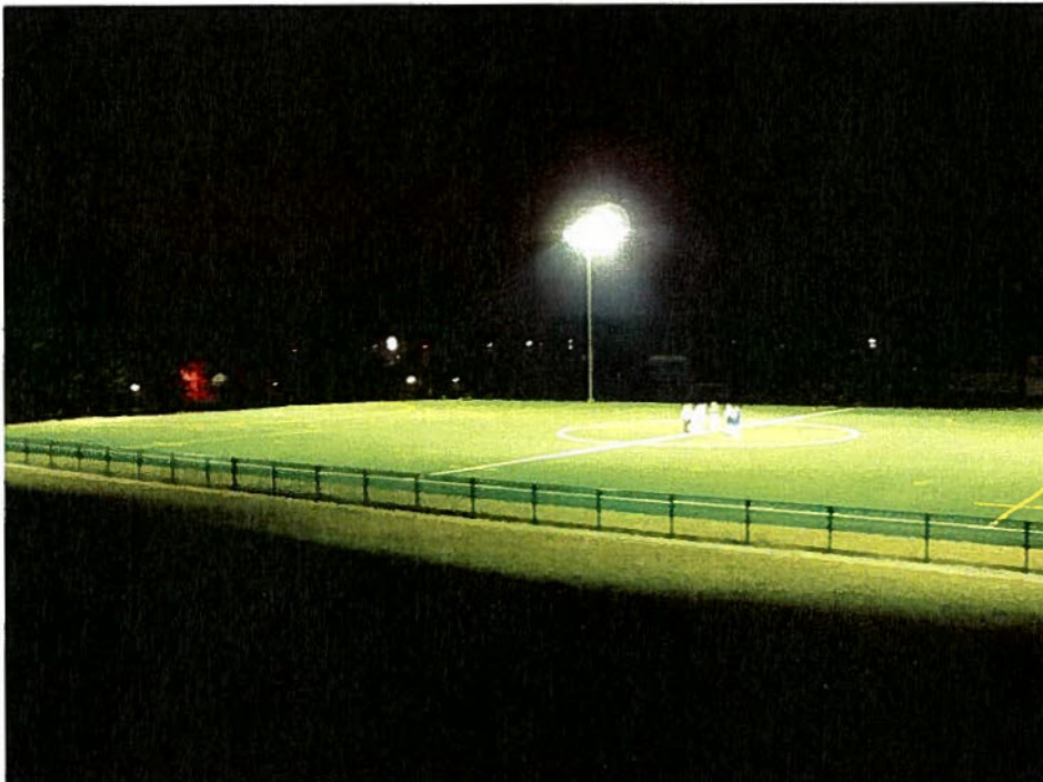
Sample Field Lighting with Low-Spill Technology at Minnie Howard Field
