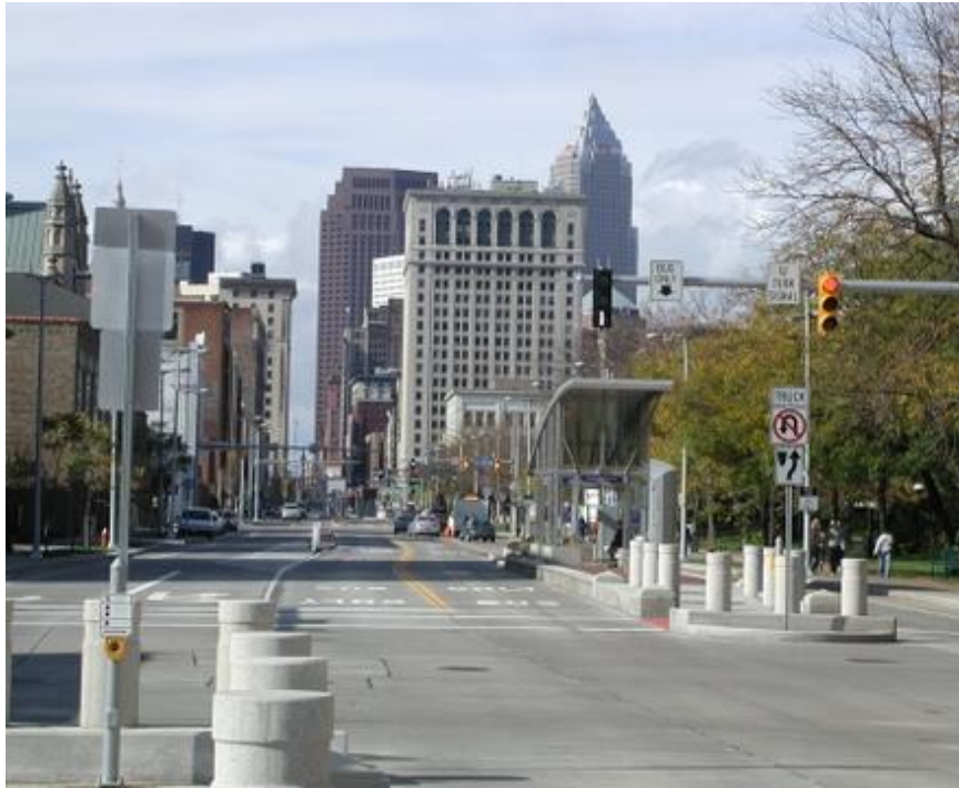
Healthline BRT runningway, Cleveland (Ohio)
