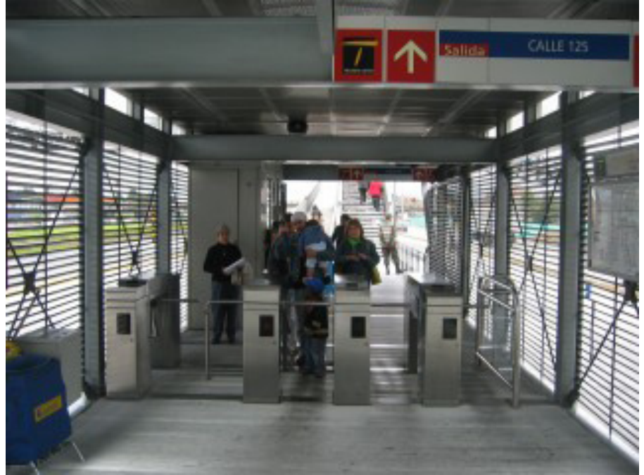
Station/stop structure for TransMilenio (Bogota, Colombia)
