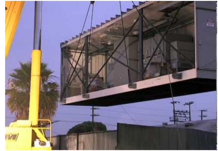
Traction power transformer, unknown location
