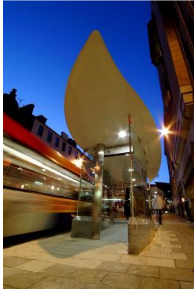
Bus shelter, Scotland (England)
