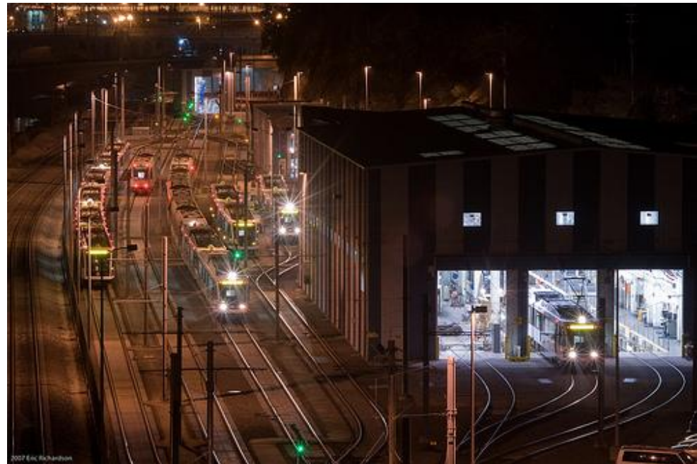
LA Metro LRT storage and maintenance yard, Los Angeles (California)
