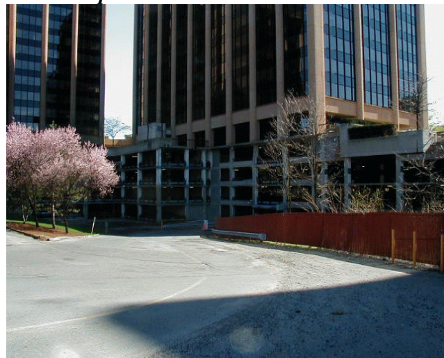
View of Exposed Parking Decks
