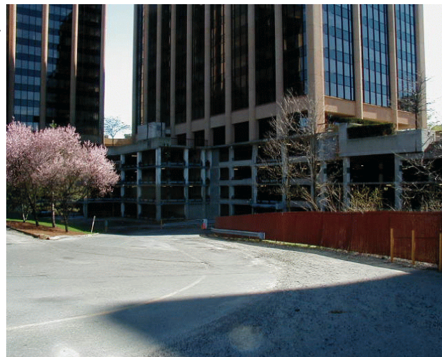
View of Exposed Parking Decks
