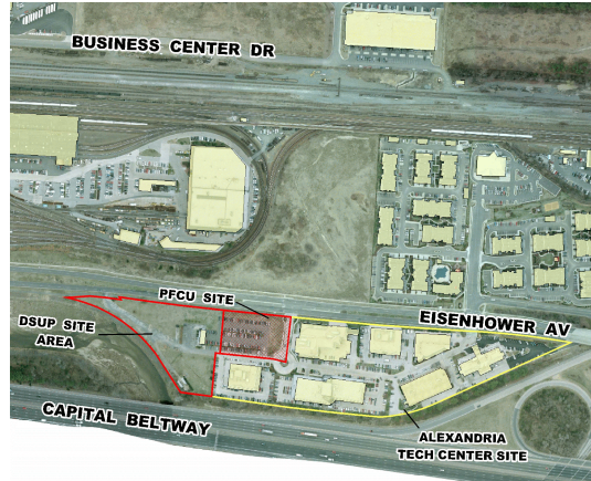
Aerial View - Alexandria Tech Center
