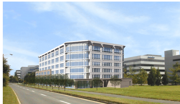
Northwest Elevation View Showing Screened Parking
