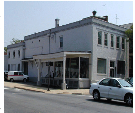
Figure 7 - Building to the East
