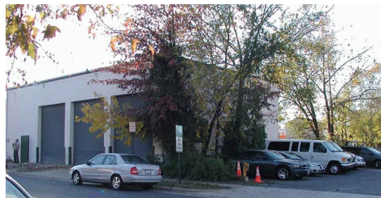
Existing site conditions
