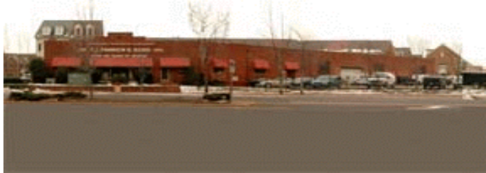
Adjacent office building
