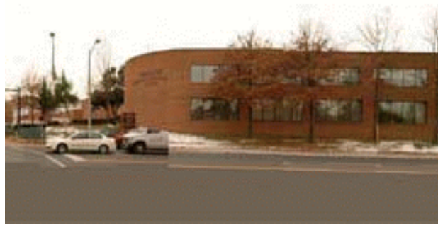
Adjacent commercial building
