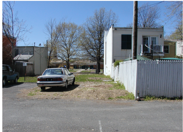
View of rear of 219 N. West St. from Alley
