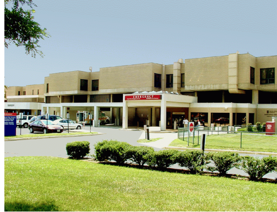
Existing Emergency Room Entrance
