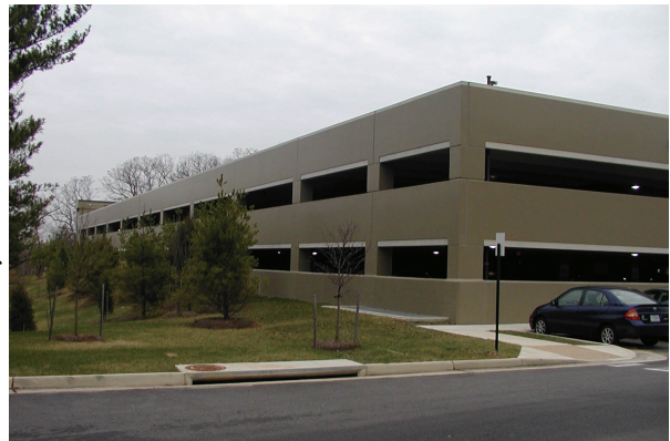
New Parking Structure
