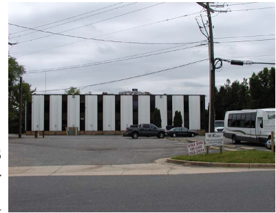
Existing On-Site Office
