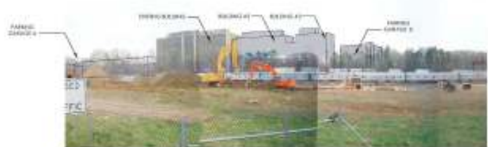
NORTH VIEW OF SITE (PHOTO VIEW #1)
