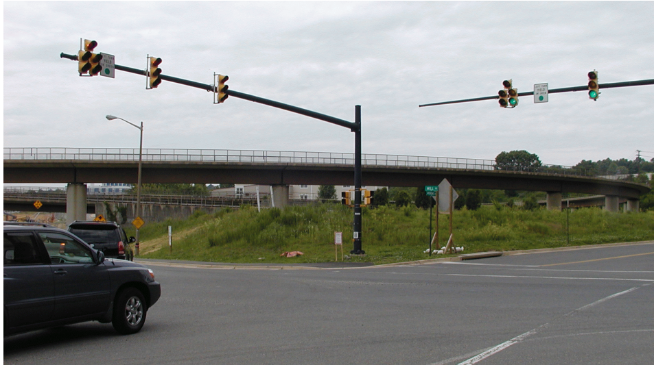
View of Site from the Mill Road and Andrews Lane Intersection
