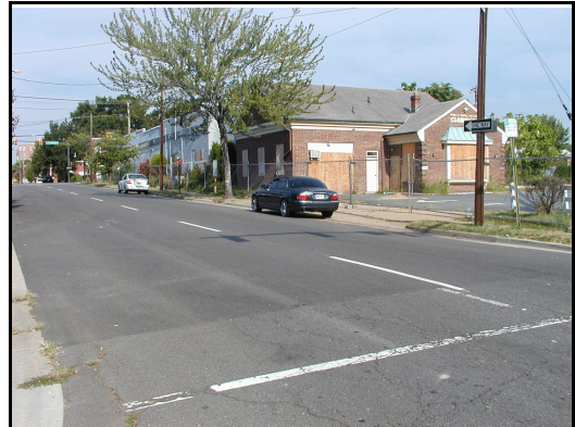
Montgomery Street Parking
