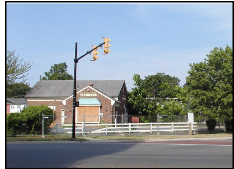
Site from Washington Street
