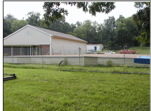
Existing Foundation along Fillmore Avenue
