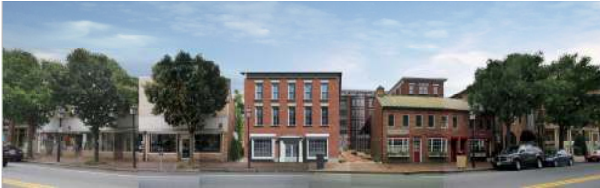
Figure 9: King Street Building Montage
