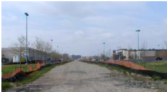
Figure 2. Potomac Avenue/Temporary Hauling Road
