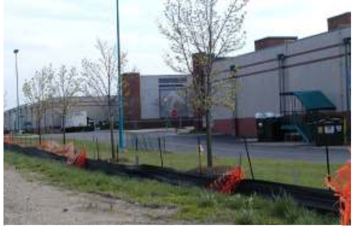
Figure 6. View of Service Area behind Retail Center
