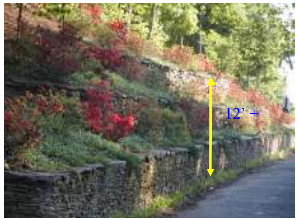
Figure 7: Retaining Walls at Pickets Ridge
