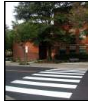
Figure 11. High-visibility Thermoplastic Crosswalk
