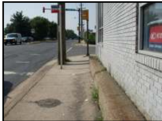
Figure 10. Example of a Narrow Sidewalk on the west side of Route 1
