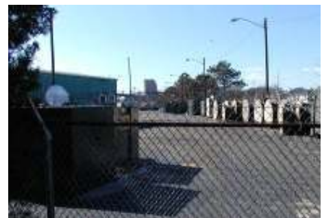
Fig. 24: WEST GLEBE – View of Dominion Power from site
