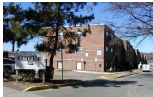
Fig. 21: WEST GLEBE – View of Existing Bldg from W. Glebe Rd.
