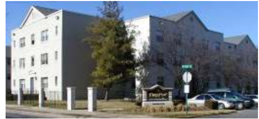
Fig. 20: WEST GLEBE – Adjacent Kingsport Apartments
