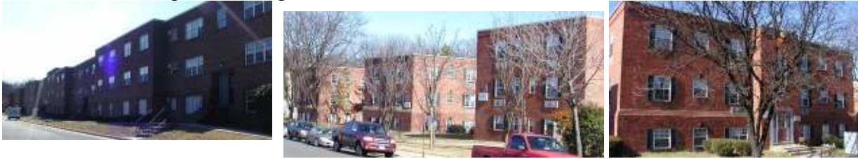
Fig. 10: EXISTING BUILDINGS – West Glebe, Old Dominion East, Old Dominion West.
