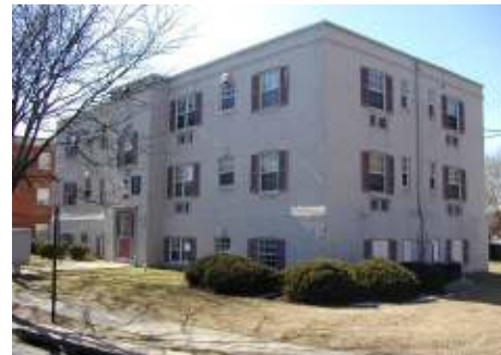
Fig. 17: OLD DOMINION WEST – Ex. Building on Corner at 3910 Old Dominion Blvd
