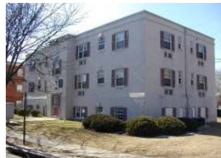
Fig. 4: OLD DOMINION WEST – Existing Building on Corner
