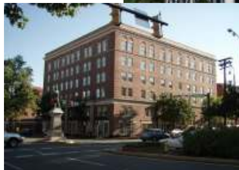
Figure 3: Washington Street - Buildings of Historic Architectural Merit
