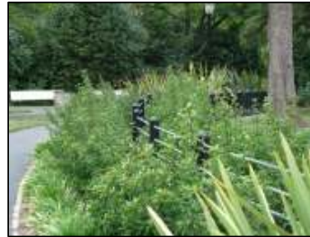
Figure 7. Post and Cable Security Fencing
