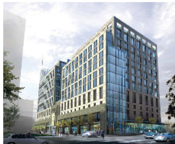
Figure 2. Block P west (765 John Carlyle St.), as viewed from Eisenhower Ave.
