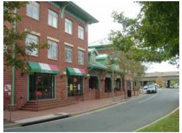
Streetscape enhancements can add value to existing ground-floor retail along Braddock Road.
