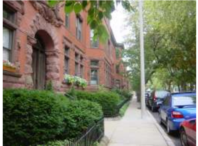
This building incorporates high quality brick with heavier masonry materials at ground level.
