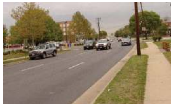
Route 1 is a principal gateway street in the Braddock Metro neighborhood.
