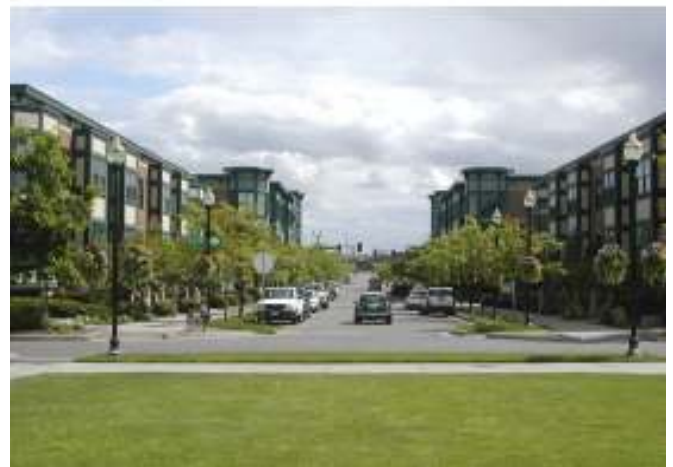
Consistent building edges flanking the street, together with street trees of consistent height and/or planting pattern, help define the street as a three-dimensional public space.
