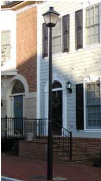
Dominion Virginia Power colonial light fixtures
