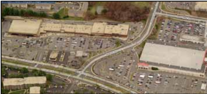
Strip shopping centers and big-box stores are typically one story with surface parking.
