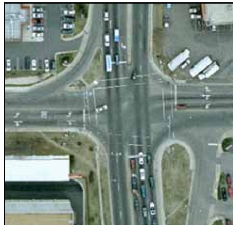
The intersection of Van Dorn Street and Pickett Street shows the gauntlet of high-speed right-turn lanes, large curb radii and driveways that challenge pedestrian travel.
