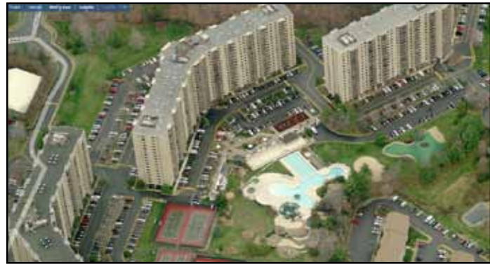
High-rise apartment and condominium building type.
