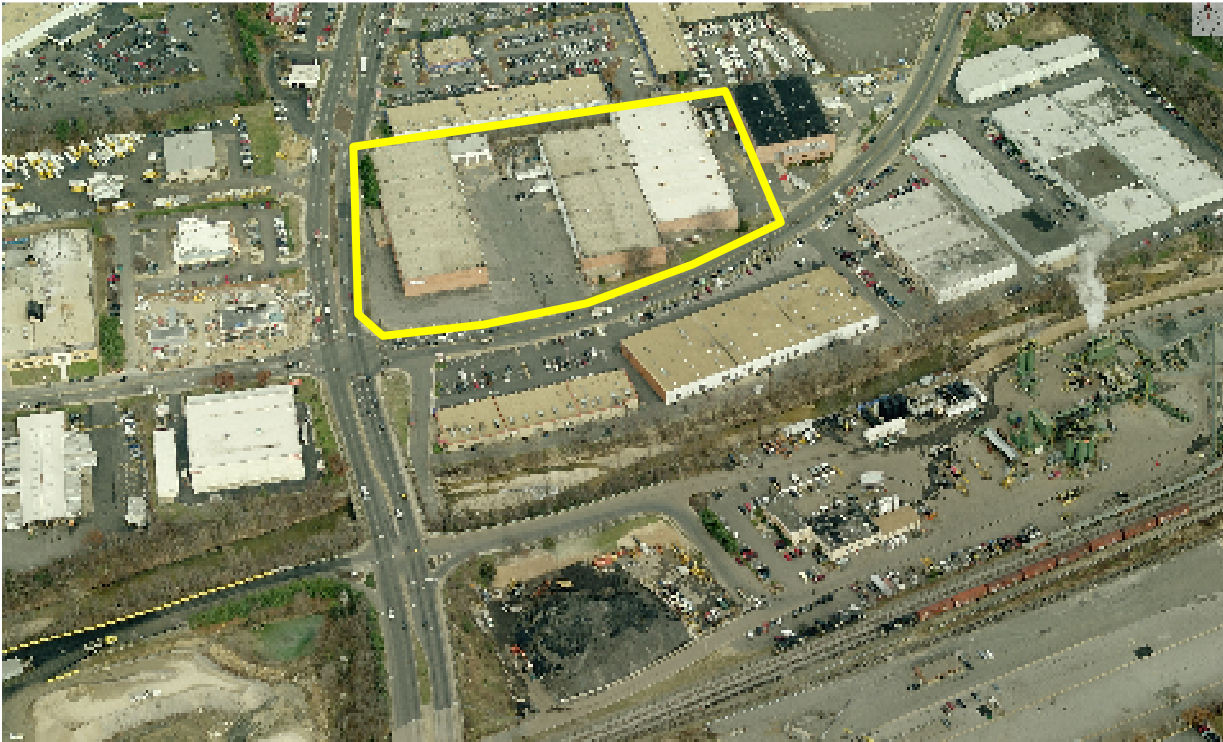
Figure 11: View of Landmark Gateway site looking north
