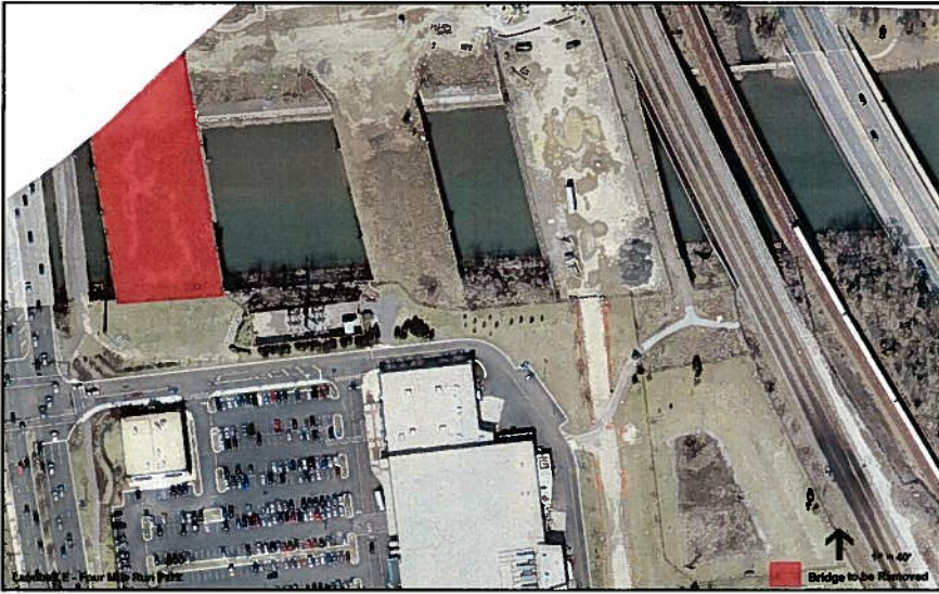
Figure 1: Site Aerial - Bridge "B"
